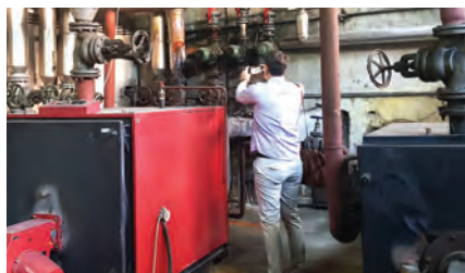
Inspection to planned locations for improving heating systems.
